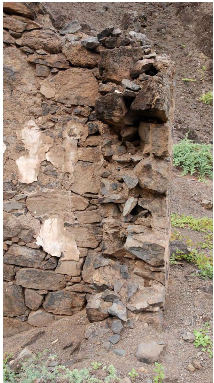
The Mud Mortar And Plaster Of This Wall Have Been Skimmed Over With A Fine White Lime
