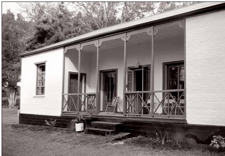
FIGURE 20: Integral verandah – Olive Cottage
