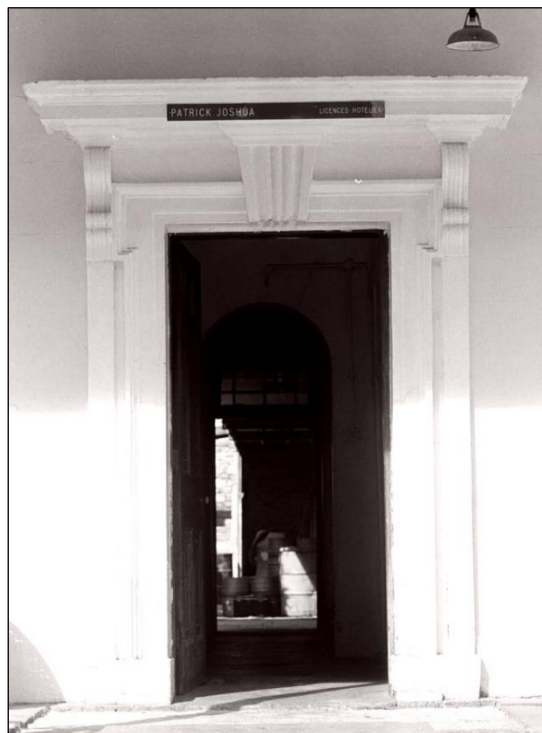
FIGURE 21: Details: door surrounds, Consulate Hotel
