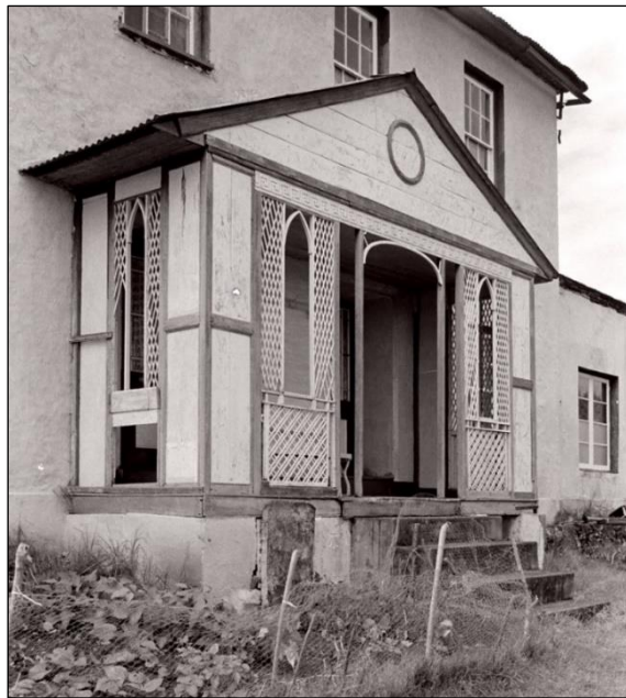
FIGURE 18: Porch – Alarm House
