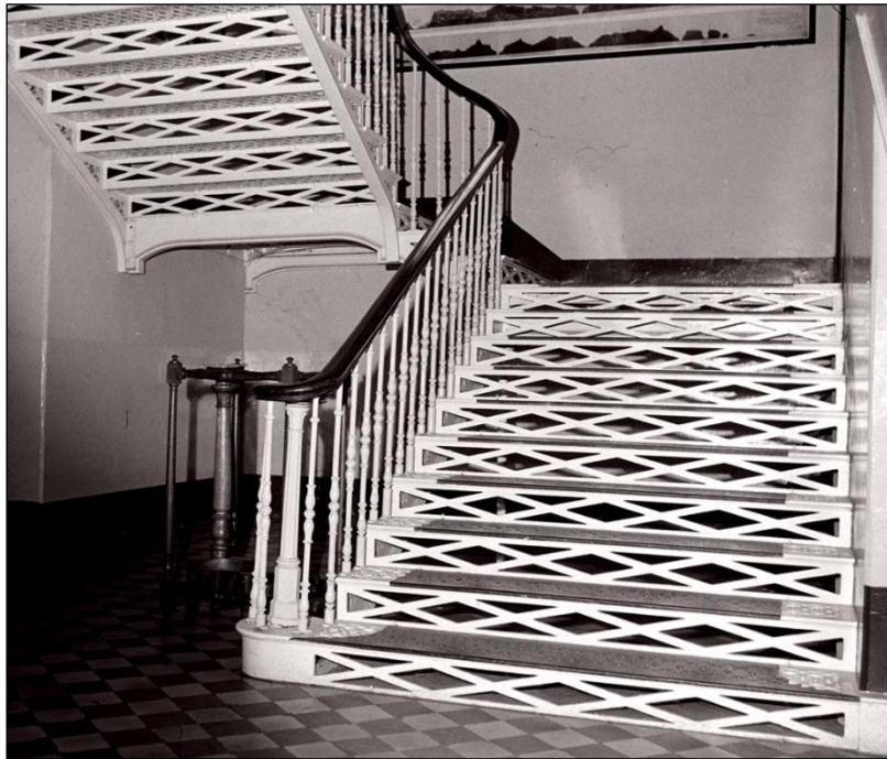
FIGURE 11: Cast iron staircase – The Castle
