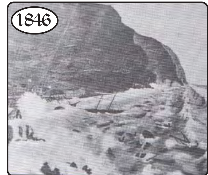
1846 Heavy seas and rollers in February greatly damage the sea defence wall and the Wharf and demolish 13 ships.
